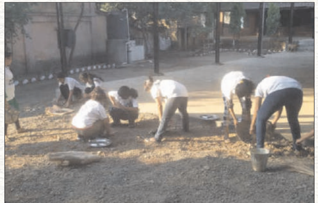
Leveling of school courtyard in Dahanu
